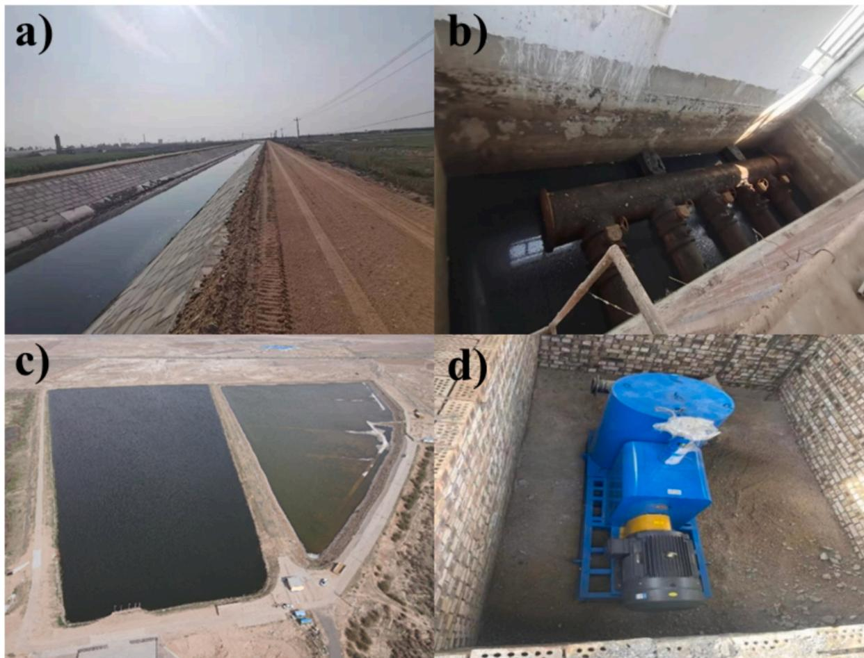
Fig. 4. (a) The stormwater channel; (b) The rainwater pump; (c) The rainwater reservoir; (d) The rainwater reuse pump.
